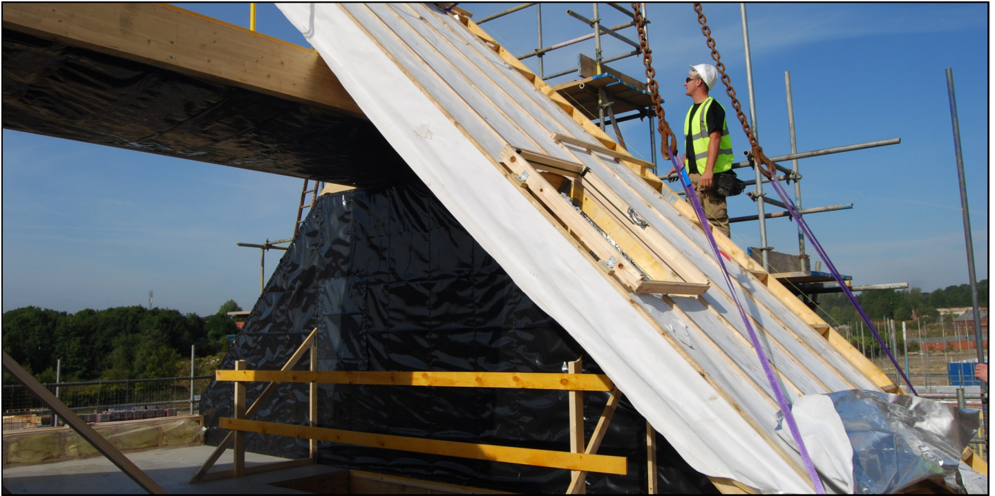
Pre-Insulated, felted and counter battened offsite, the X-Rafter cassettes are craned into position.
