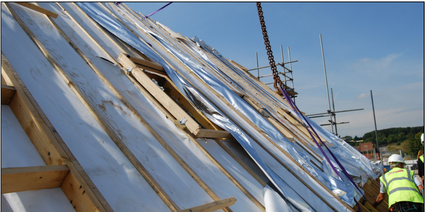
The Posi-Joist cassette floor and the structural ceiling cassettes form two safe working platforms providing that the appropriate harnessing is worn by the installation team.
